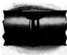
FIG. 64. — Stove-pipe Joint.
